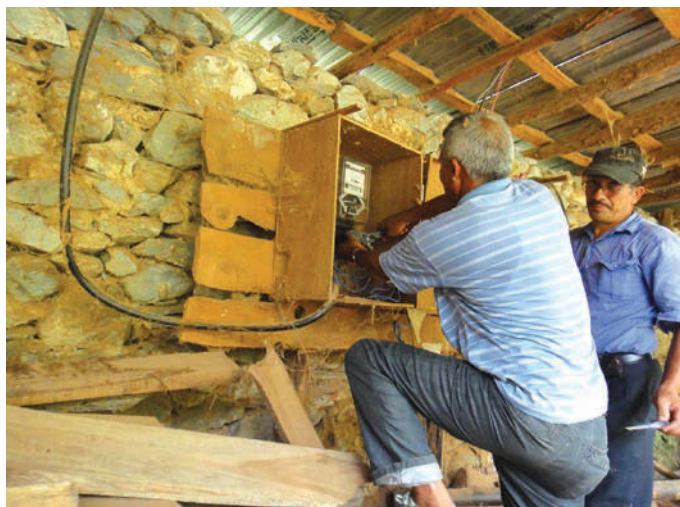
Meter resealing being done by NEA Employee
