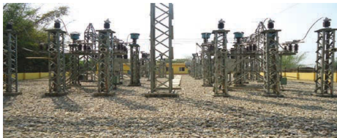
Completed Dhulabari 33/11 kV, 6/8 MVA Substation
