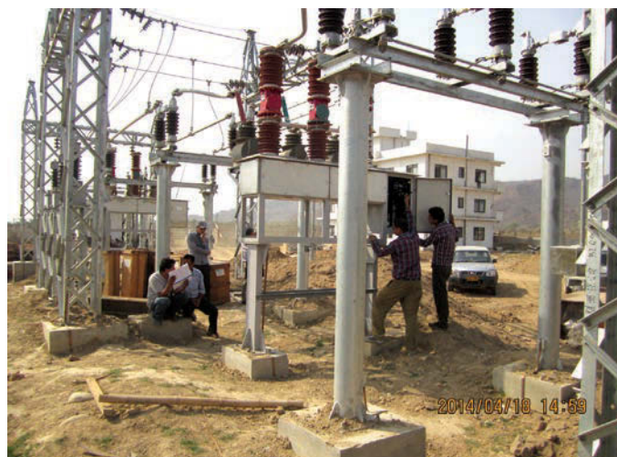
Construction Works of 33 kV S/S
