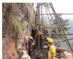
Core drilling at Tanahu HEP
