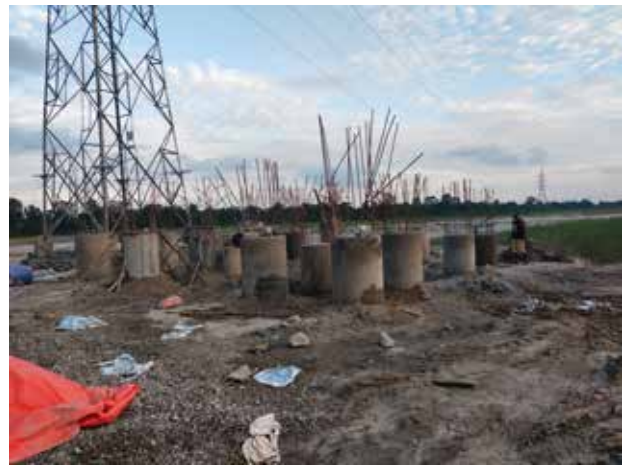
Tower protection work, duhabi-anarmani section 132 kV transmission line tower no. 37 (Lohandra Khola)
