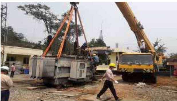
15 MVA , 132/33 kV Power Transformer Replacement Work at Damauli Substation
