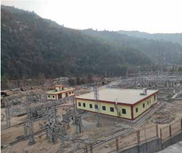
33 kV switchyard, control building, 132 kV Switchyard & TL Towers
