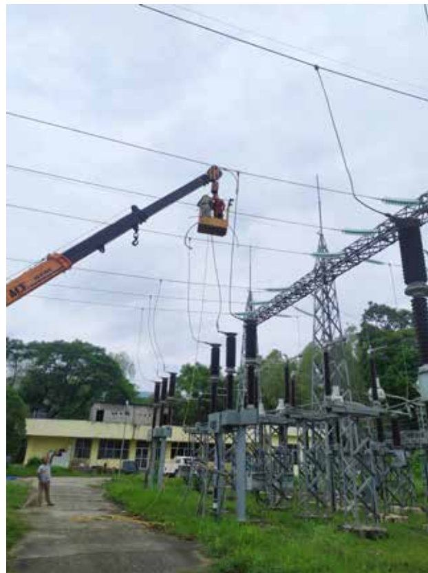
Conductor Maintenance of KG 1 & 2 Circuit
