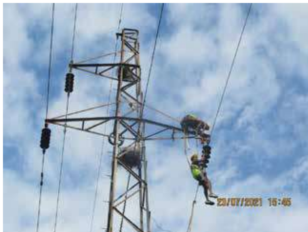
Conductor Stringing Works
