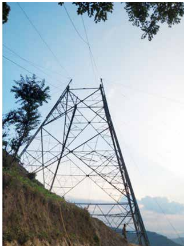
Tower erection works at AP 30/0 for Bahrabise-Kathmandu 400 kV transmission line
