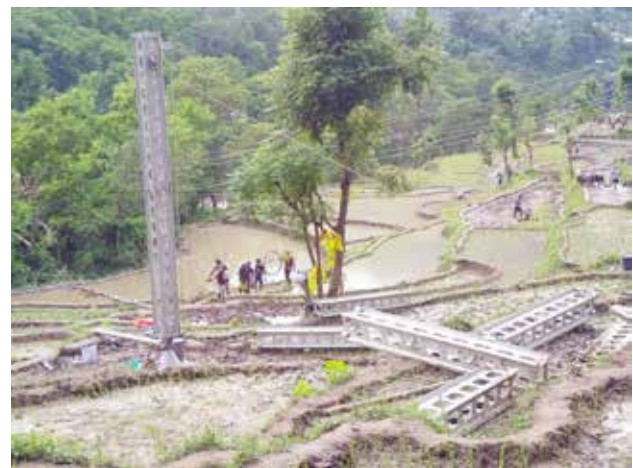
Transportation and erection of ERS components
