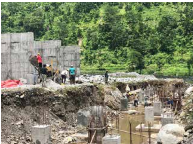
Foundation Work with Fire Walls under construction
