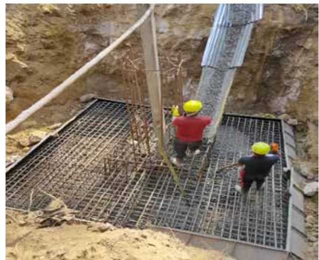
Pad Concreting of Leg A of AP-34D of Udipur-Bharatpur 220 kV Transmission Line Project
