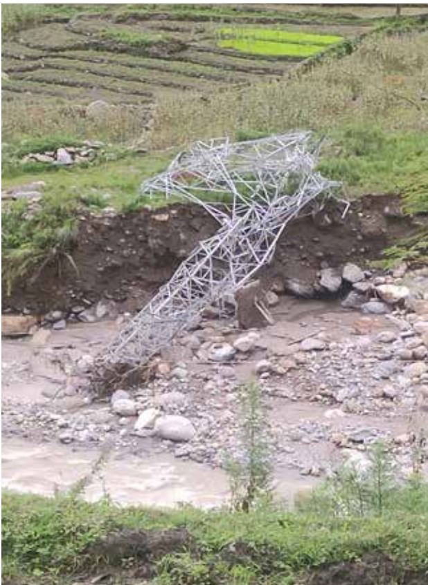
Collapsed Tower
