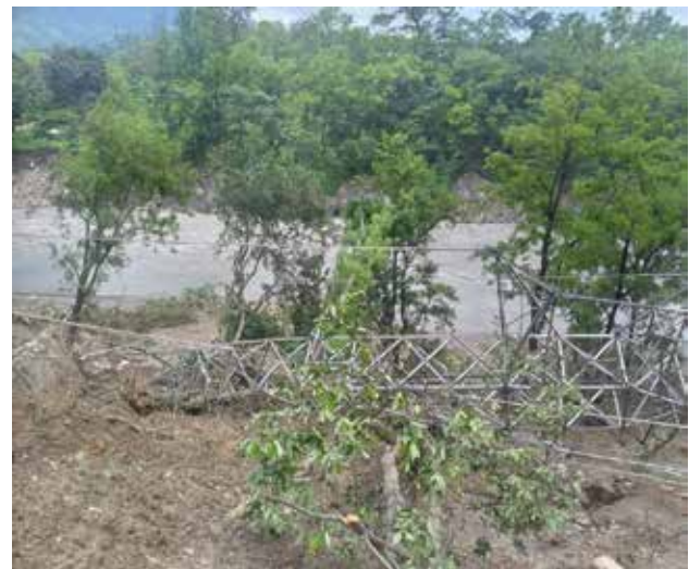
TN-09 Collapse due to Landslide
