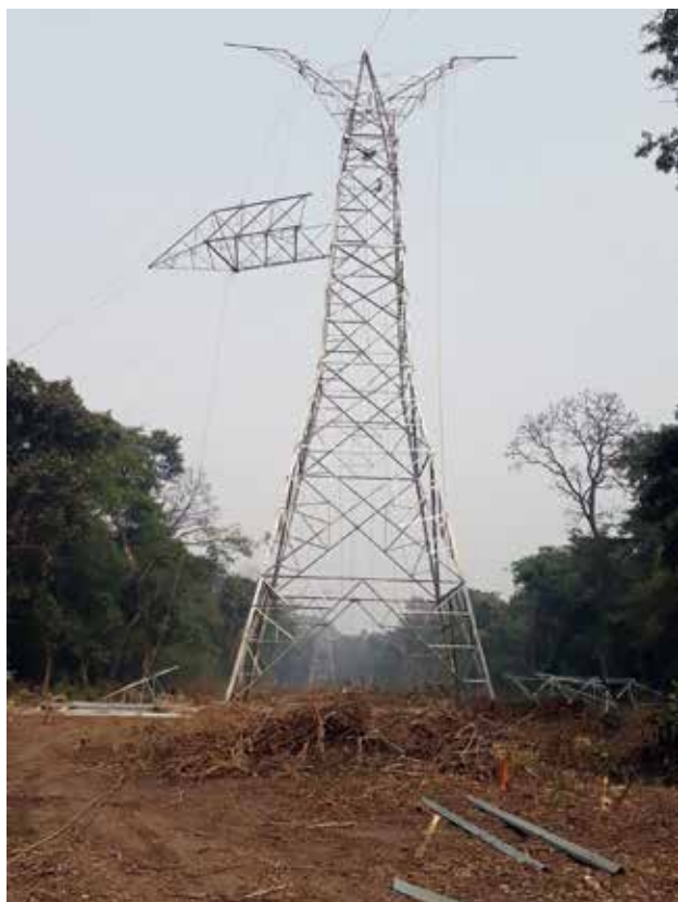
400 kV Tower Erection Works
